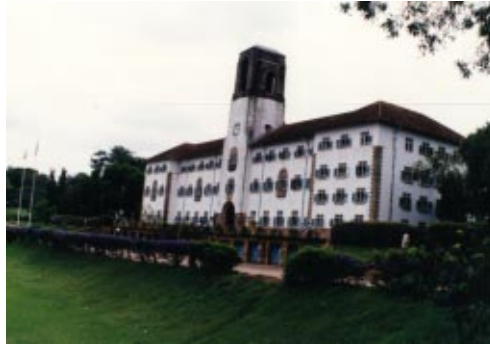
Figure 11: Makerere Main Building, Kampala. Source: Private Collection
