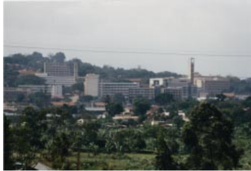
Figure 16: Kampala Skyline - Uganda Parliament Building to the right, obscured by other buildings.
