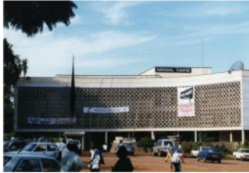
Figure 20: National Theatre and Cultural Centre, Nakasero, Kampala. Source: Private Collection.
